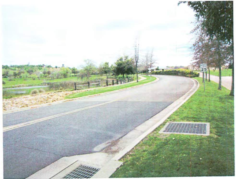
Near Roundabout, Looking Toward Realty Office
